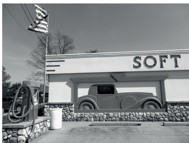
Figura 12. Lake Orion, Michigan, Car Wash, 120 W. Shadbolt Street
